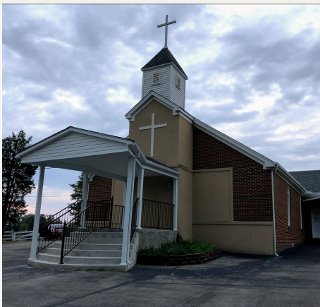
Sept/2018 Newly Renovated Entrance
